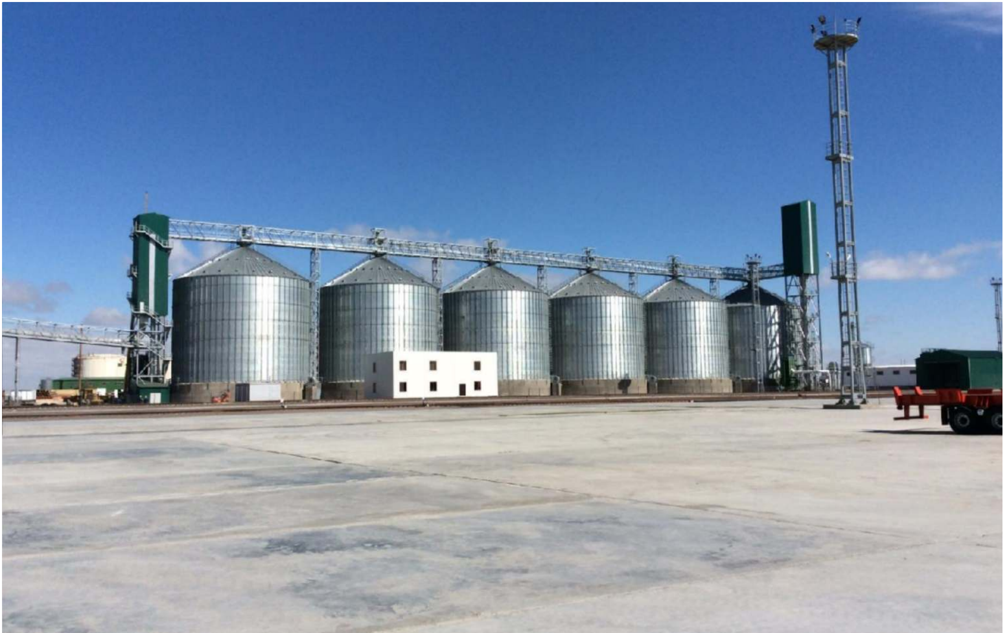
2015 AKT - KAZAKHSTAN: 6 silos mod. 27,50/18 - Total capacity: 62.000 T
