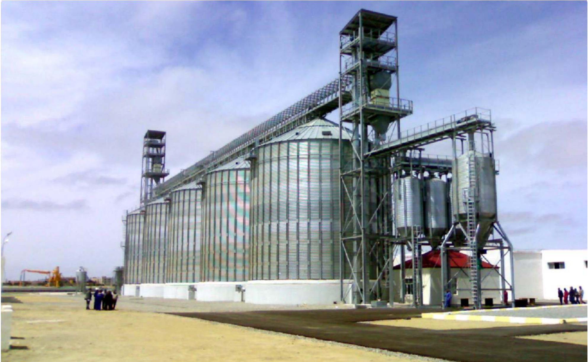
2007 BAKU - AZERBAIJAN: 5 silos mod. 16,81/14 – Total capacity: 15.000 T
