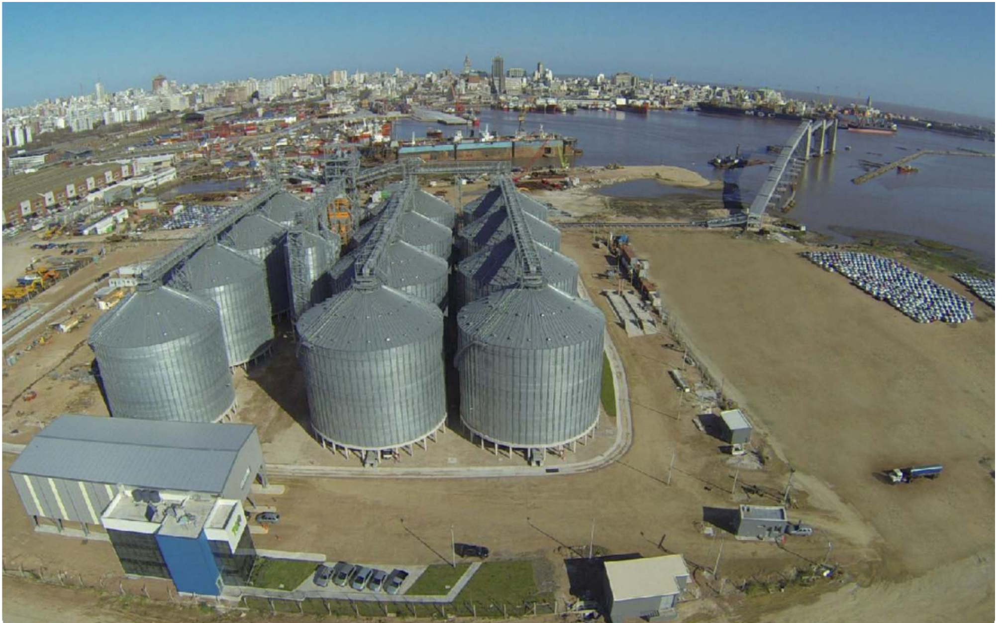
2015 OBRINEL - URUGUAY: 12 silos mod. 27,50/17 - Total capacity: 121.000 T
