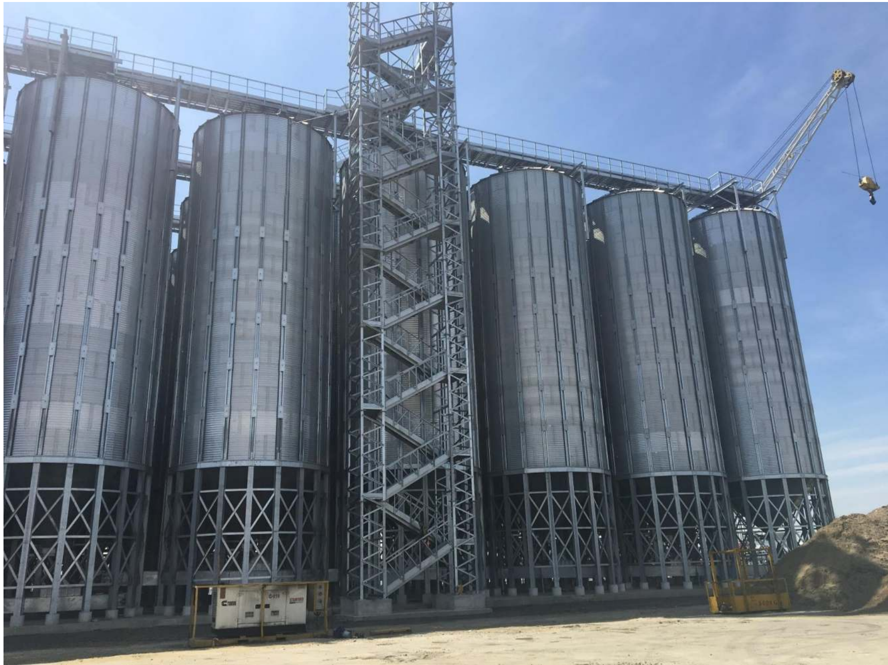
2018 PORT OF ANTWERP - BELGIUM: 37 hopper silos 45° mod. 07,64/16 Total capacity: 25,750 T
