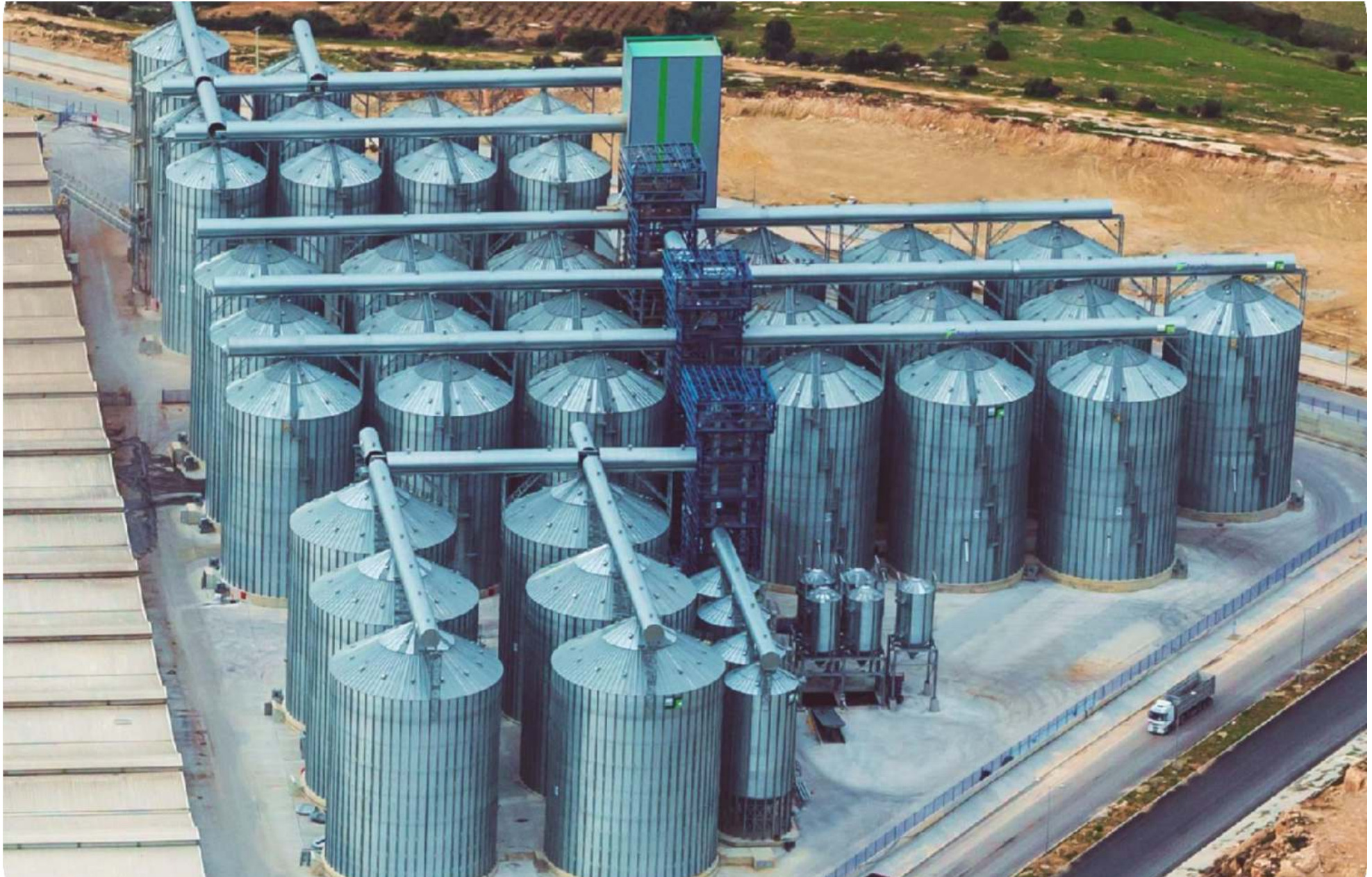
2013 TIRYAKI - TURKEY: 19 silos mod. 18,33/22 – 11 silos mod. 14,51/22 – 27 truck load silos mod. 4,65/6 – 6 silos mod. 21,39/22 – Total capacity: 200.000 T
