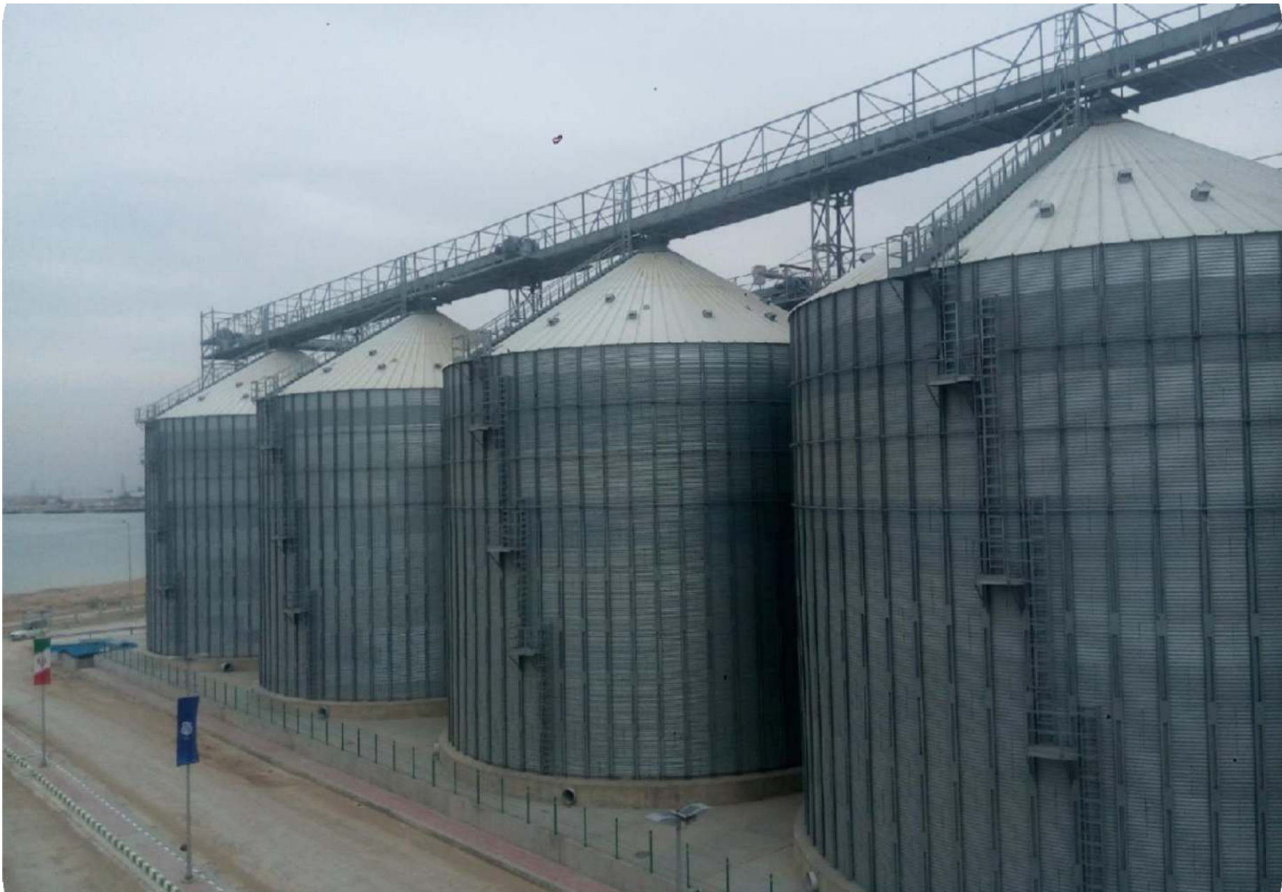
Under construction NKF - IRAN: 48 silos mod. 24,45/17 - Total capacity : 367.000 T
